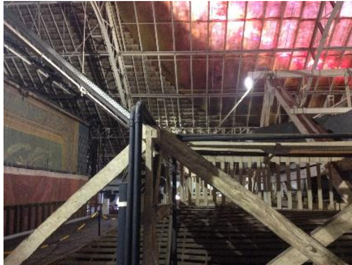
Figure 2.11 Light reflector at the first part of the warp.
